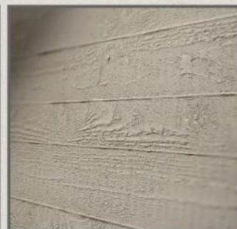
122E timber formwork
